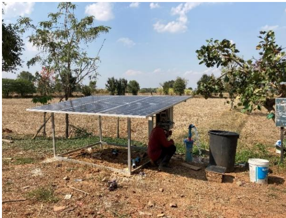
Fig. 7 The artesian well pumps water with solar cells which farmers operate by themselves
